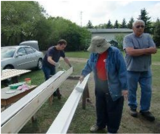
Mark Fidelak and Ev Chimboryk priming siding while Les Gamel supervises.
