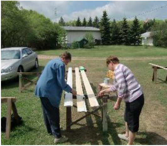
Ev Chimboryk and Linda Flory applying primer to newly milled siding.
